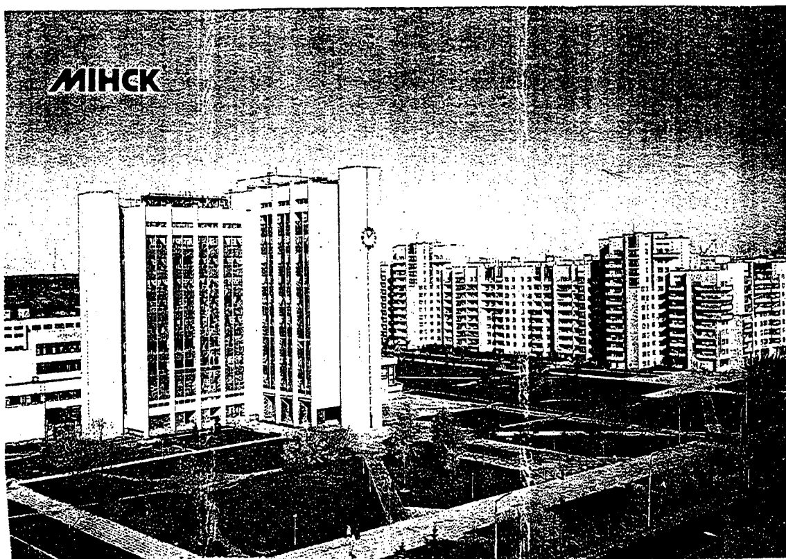
Minsk. An office building
